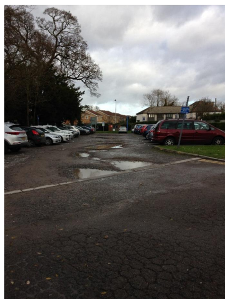
Internal Site Road
