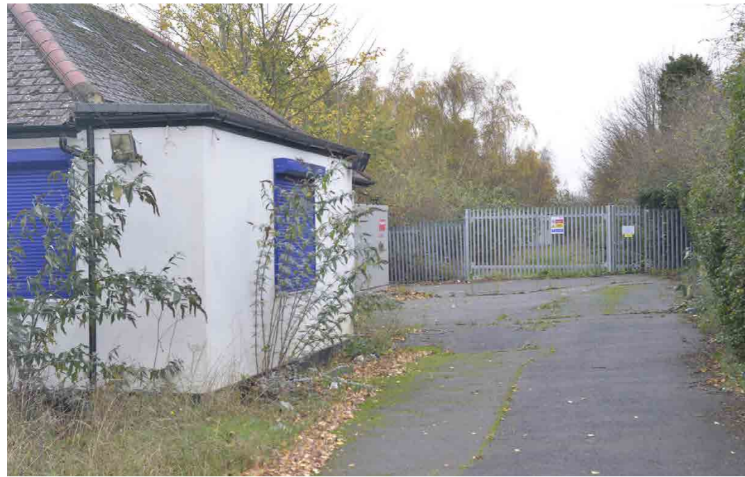
Viewpoint 4.7. Looking northwest
