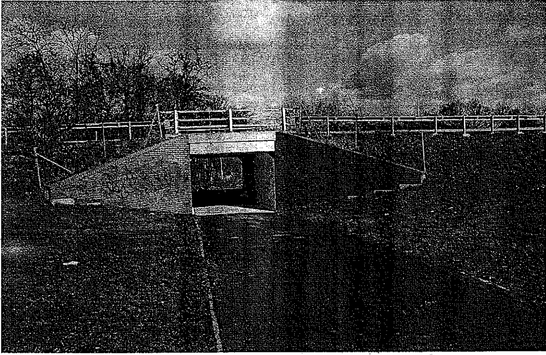
Plate 3: Underpass access to the Freezeland Covert, North Hillingdon.
