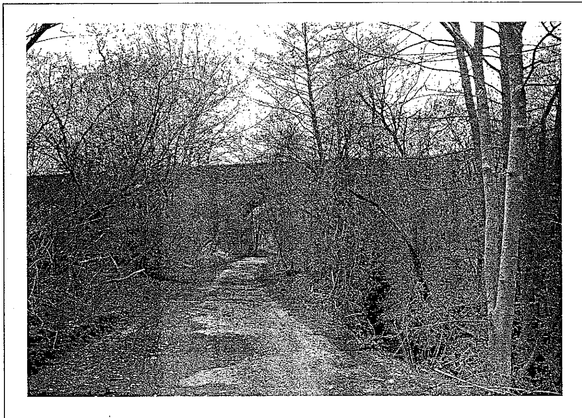
Plate 4: Railway overpass through Fray's Valley Nature Reserve, Ickenham
