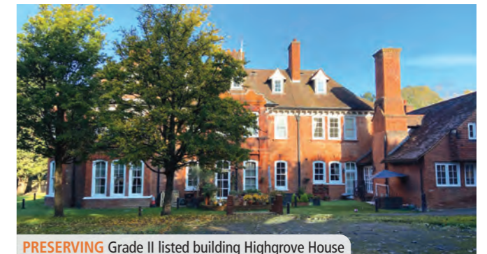
PRESERVING Grade II listed building Highgrove House
